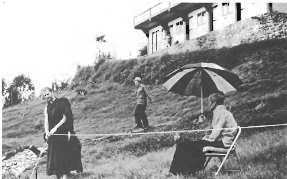
Supervising construction at Sonada, 1981
