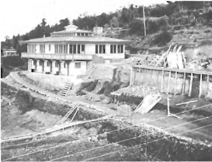
Sonada under construction
